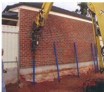
Plate B – Installation of Blade Pile
