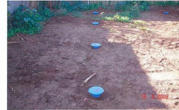
Plate C – Pile caps in place
