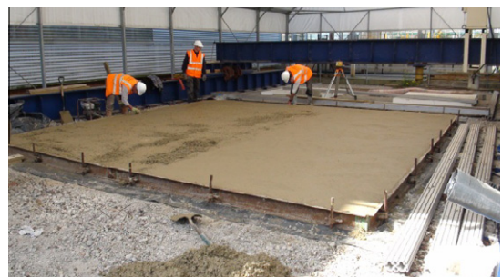
Fig. 7. Placing concrete at different stages.
