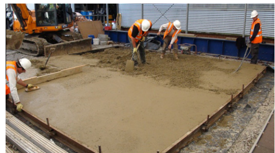
Fig. 6. Placing concrete at different stages.
