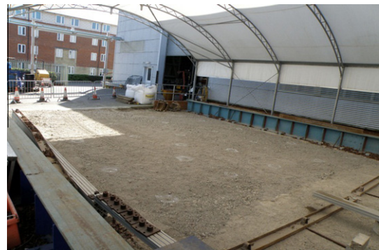
Fig. 5. Completed ground work for the required CBR value.
