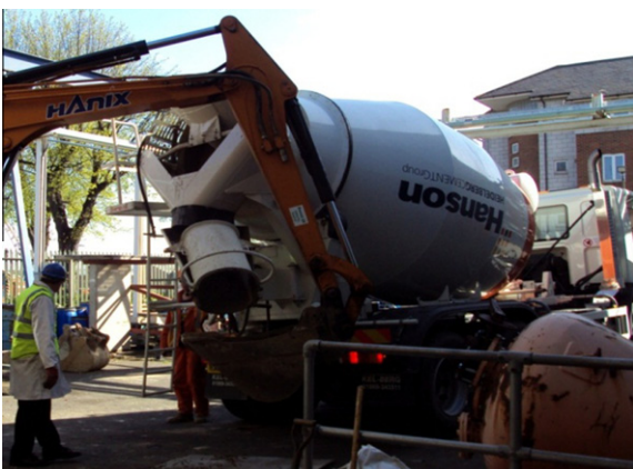
Fig. 3. Ready mixed concrete supplied by Hanson UK.
