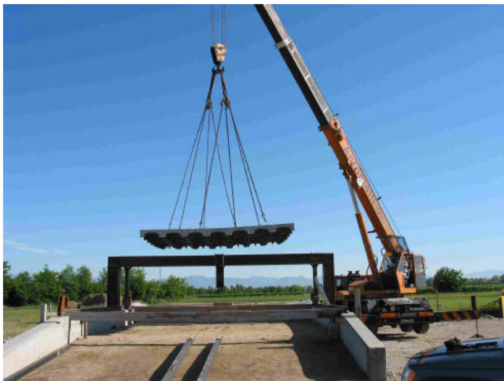
Fig. D.9: Lifting of concrete tests
