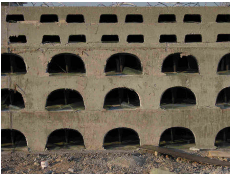
Fig. D.6 Frontal detail of concrete tests
