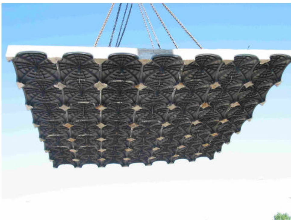
Fig. D.10: Detail of concrete tests lifting
